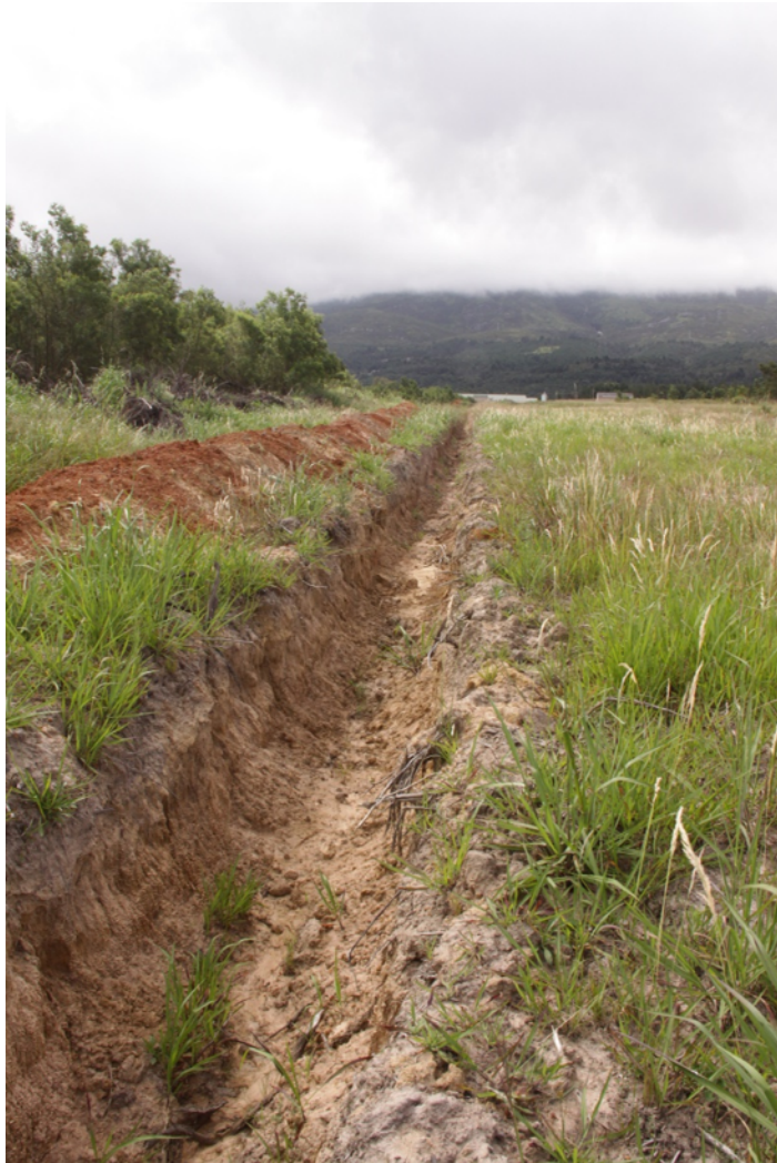
Trenching for storm water control along the western boundary of the site
